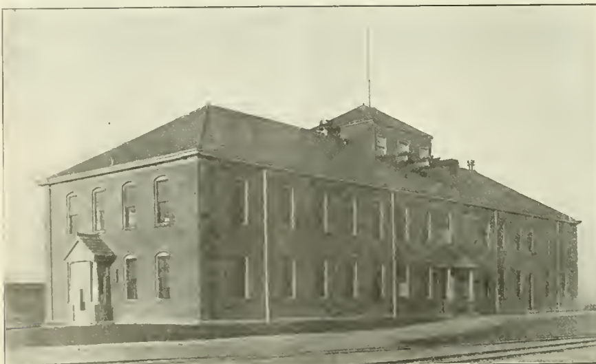
OFFICE BUILDING AT THE OMAHA SHOPS OF THE UNION PACIFIC.
